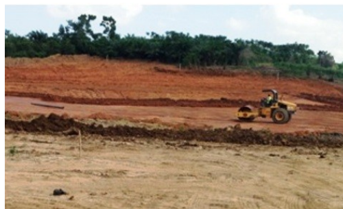
PIC 5: EARTHWORKS AND SOIL STABILIZATION CONTINUES
