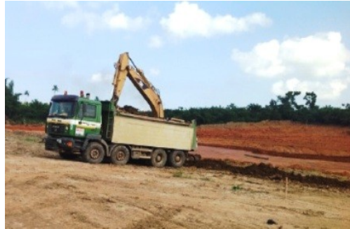
PIC 11: TIPPER TRUCK REMOVING EXCAVATED MATERIAL FROM THE SITE
