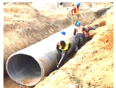
PIC 9: INSTALLATION OF CULVERT CROSSING AT THE FRONT ENTRANCE OF THE SITE
