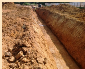
PIC 3: FRONT DRAIN EXCAVATED WITH SIDES BEVELED
