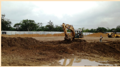
PIC 1: EARTHWORKS TO STABILIZE THE SITE BY EXCAVATING UNSUITABLE SOIL IN PREPARATION FOR LAYING OF SUB-BASE
