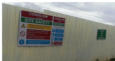
PIC 12: SITE SAFETY SIGNS HAVE BEEN PUT UP ACROSS THE ENTIRE SITE TO ENSURE THAT WORKERS AND VISITORS HAVE A VISUAL REMINDER OF SAFETY RULES DURING CONSTRUCTION
