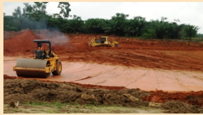
PIC 2: FILLING AND COMPACTING LOW WATERCOURSE AREAS WITH GRANULAR HARD-CORE MATERIAL
