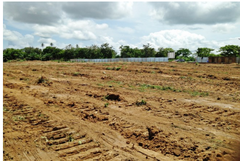
FIG 6: CLEARING OF VEGETATION AND TOP SOIL CONTINUES, AFTER WHICH CLAY SUB-LAYER WILL BE EXCAVATED AND REMOVED FROM SITE, TO BE REPLACED BY COMPACTED LATERITE FILL MATERIAL
