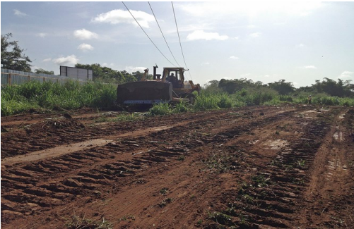
FIG 5: DEVELOPMENT BEGINS WITH CLEARING OF THICK VEGETATION FROM SITE
